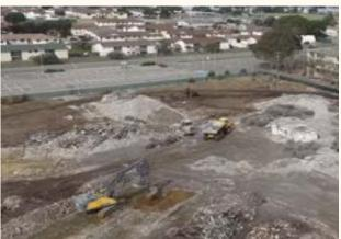
Challenges Faced: The 3-story Star barracks building was next to Job corps an active building AMPCO employed a structural engineer to provide an engineered structural demolition and a site specific dust control plan then used a multiple 300 series Excavators to demolish the building safely, with no safety incidents or accidents or public property damage.
