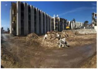
Means and Methods: The demolition scope included the implementation of SWPPP, and the complete structural demolition of the 420,000 square feet Star Barracks building and a 82,000 square feet Hanger. All building slabs, footings and underground utilities were removed. All concrete was crushed and stockpiled onsite for re-use in the grading scope, totaling 70,500 tons.
