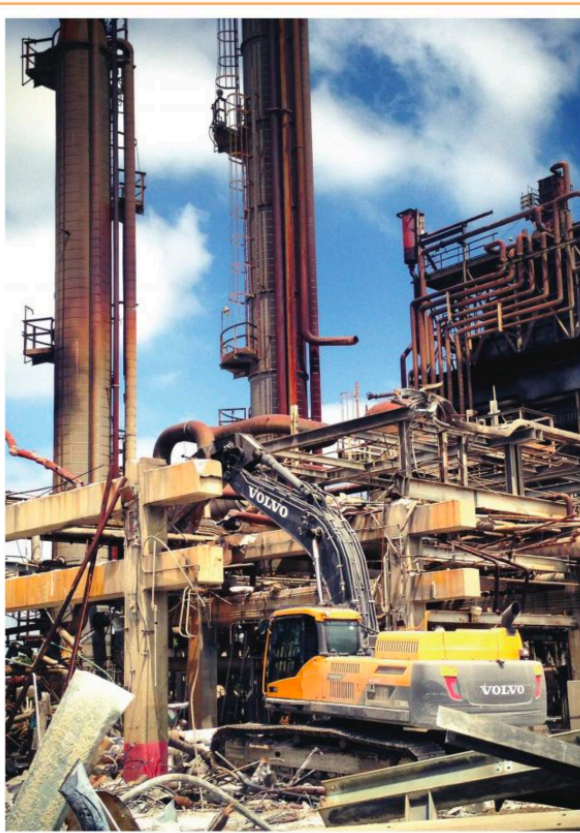
Above: AMPCO's Volvo Excavator, mounted with a LaBounty Shear, cuts up steel beams at the Lakeland Processing Hydrogen Plant in Santa Fe Springs, Calif.
