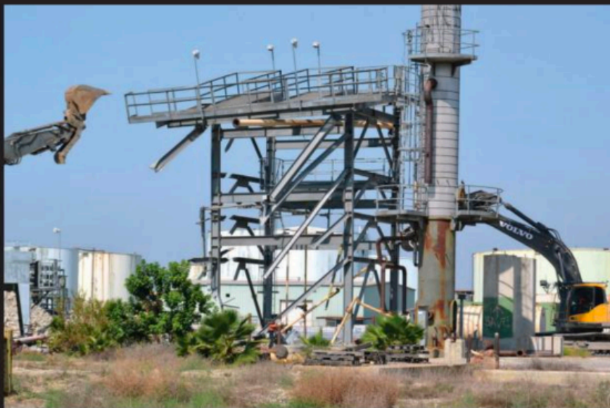
Above: Two of AMPCO's Volvo Excavators prepare to tear down a 60-foot cooling tower at the Lakeland Processing Hydrogen Plant in Santa Fe Springs, Calif.
